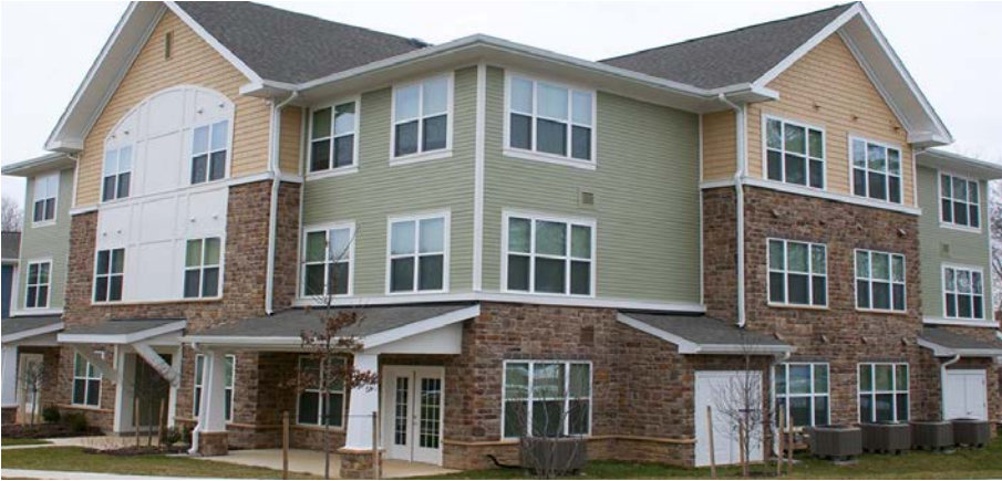
Riverwoods at Tollgate in Abingdon, MD
